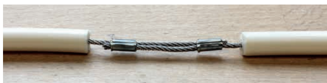
1. Join exposed reinforcement with press sleeves
